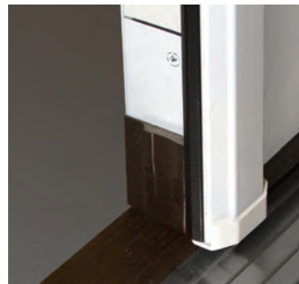
Astragal bolt penetrates threshold allowing boot to seal, creating a better barrier against the elements
